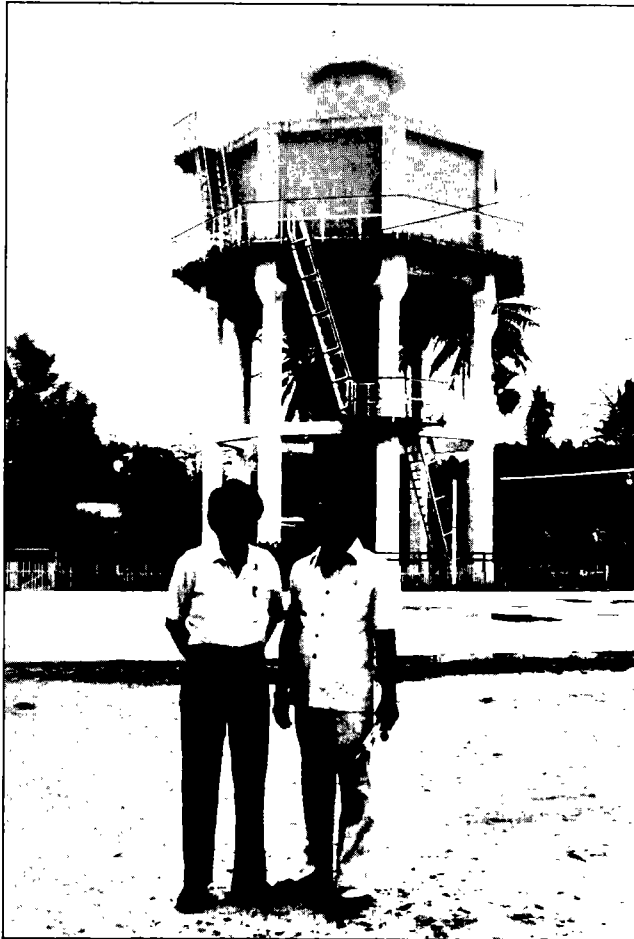
Water tower in Sigli, North Sumatra. The early 1980's saw Indonesia's water supply sector grow rapidly — most notably in the urban areas. Planning for staff increases and training therefore became urgent.
