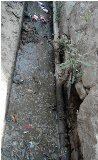
**Figure 1** Typical practice of installing drinking-water delivery pipes inside open waste and storm water channels
